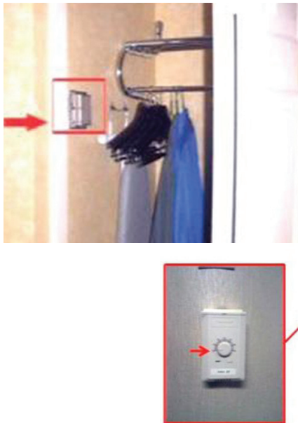
Figure 1. Optimal thermostat placement? The thermostat in the hotel room shown at left had been placed in a closet. A pillar in an airport concourse (below, courtesy of Bryan Eisenhower) had thermostats on opposing sides, set at different temperatures.
